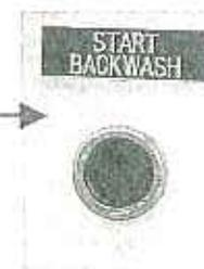
After the three filters are back online, put the dirty filter into backwash by pressing the start backwash button on the Filter Control Panel
