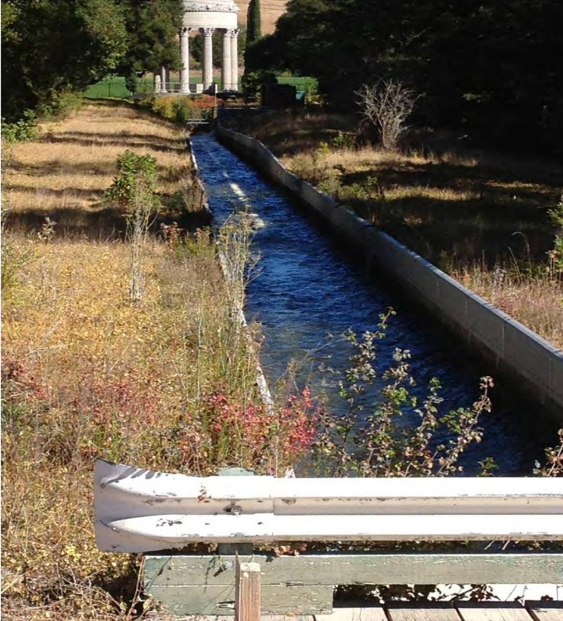
**Pulgas Release Channel (2012)** The Pulgas Release allows for system water to be added to Upper Crystal Springs Reservoir storage. Releases are not constant and vary in rate depending on the season and system-wide demand for water. (Photo: upstream view of release channel with the Pulgas Water Temple in the background.)
