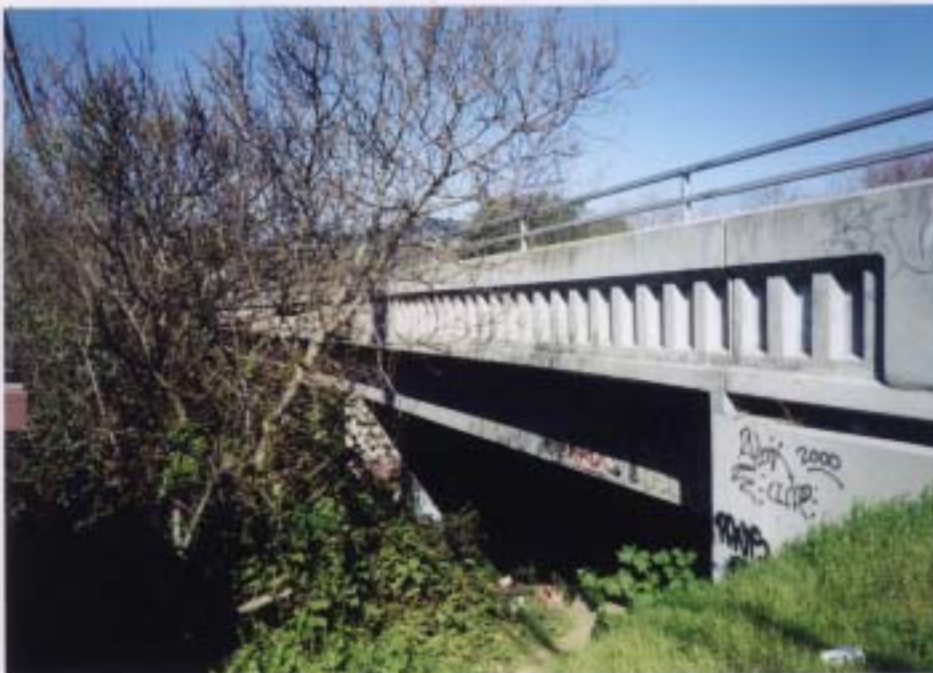
PILARCITOS CREEK BRIDGE OF HIGHWAY 1
