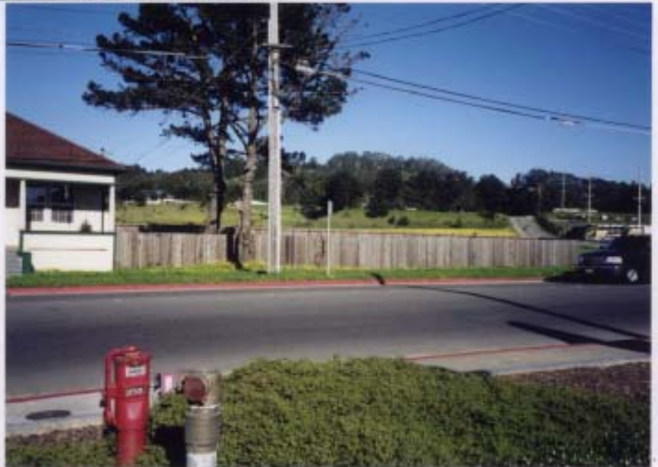
PIPELINE ROUTE ON MAIN STREET AND LOOKING EAST UP FOSTER DRIVE TOWARDS NUNES WTP
