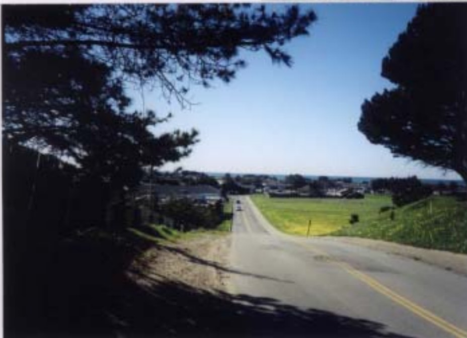
LOOKING WEST ALONG FOSTER DRIVE OF PIPELINE ROUTE TOWARDS WELL FIELD
