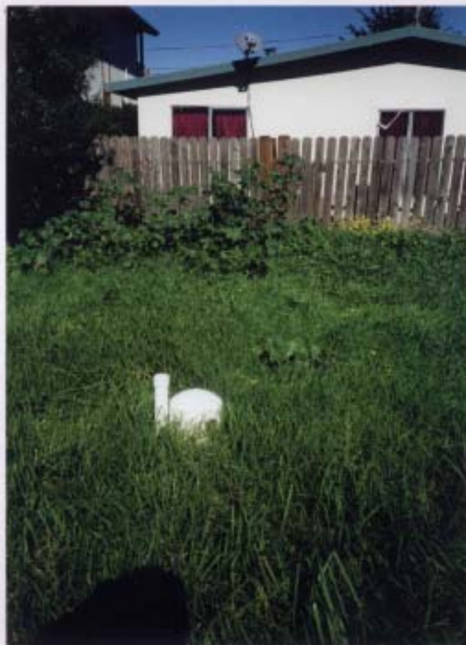
TEST WELL 2 WITH 8" PVC CAP AND RISER
