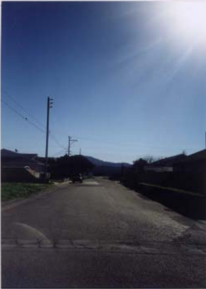
PIPELINE ROUTE ON ST. JAMES AVENUE BETWEEN CHESTERFIELD STREET AND BELLEVILLE BOULEVARD
