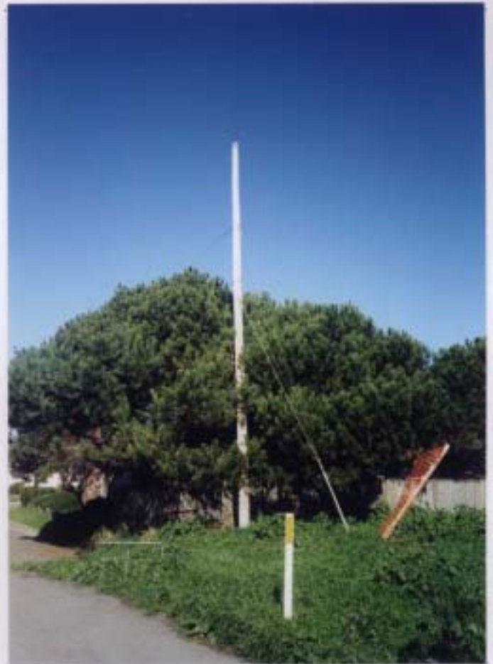
ELECTRIC SERVICE POLE ACROSS ST. JAMES AVENUE FROM TEST WELL 5
