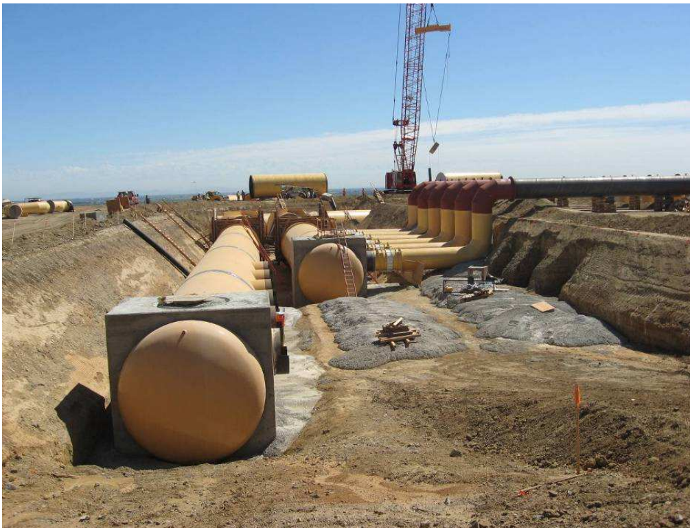
WISP Projects: The top picture is construction of the new Coast Range Tunnel Ventilation system, and the lower one is construction of the new Tesla UV treatment facility (A. Dufour).
